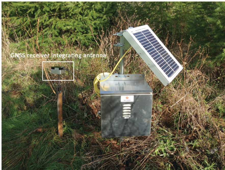
Figure 5. GNSS receiver and its power supply.
